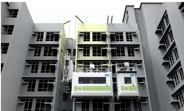
Figure 1: The visualisation shows the multifunctional modular façade-processing robot for finishing works in high-rise housing construction in Hong Kong
